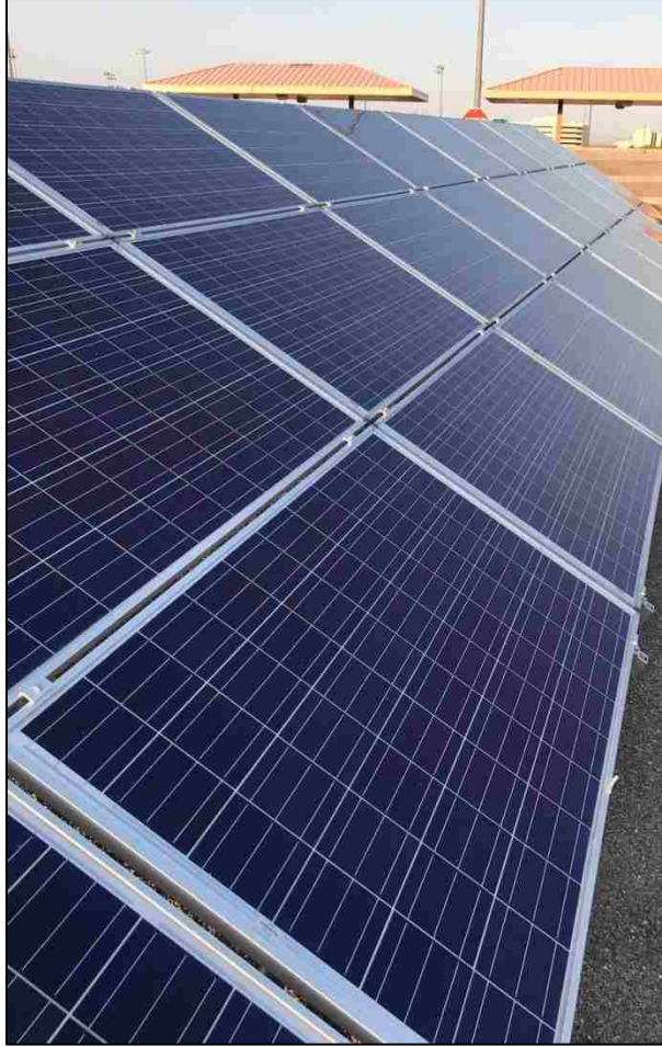
Figure 18. Clean surface after rainfall events that happened on August 2, 2017 (1.77 mm) and August 3, 2017 (1.52 mm)
